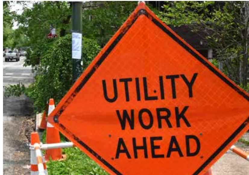
Peoples Gas work site. Credit: Author photo
